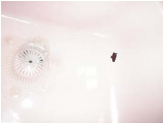
Bathroom sink basin damage penetration
